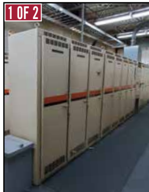
RELIANCE ELECTRIC Engineered VS Drive Units
